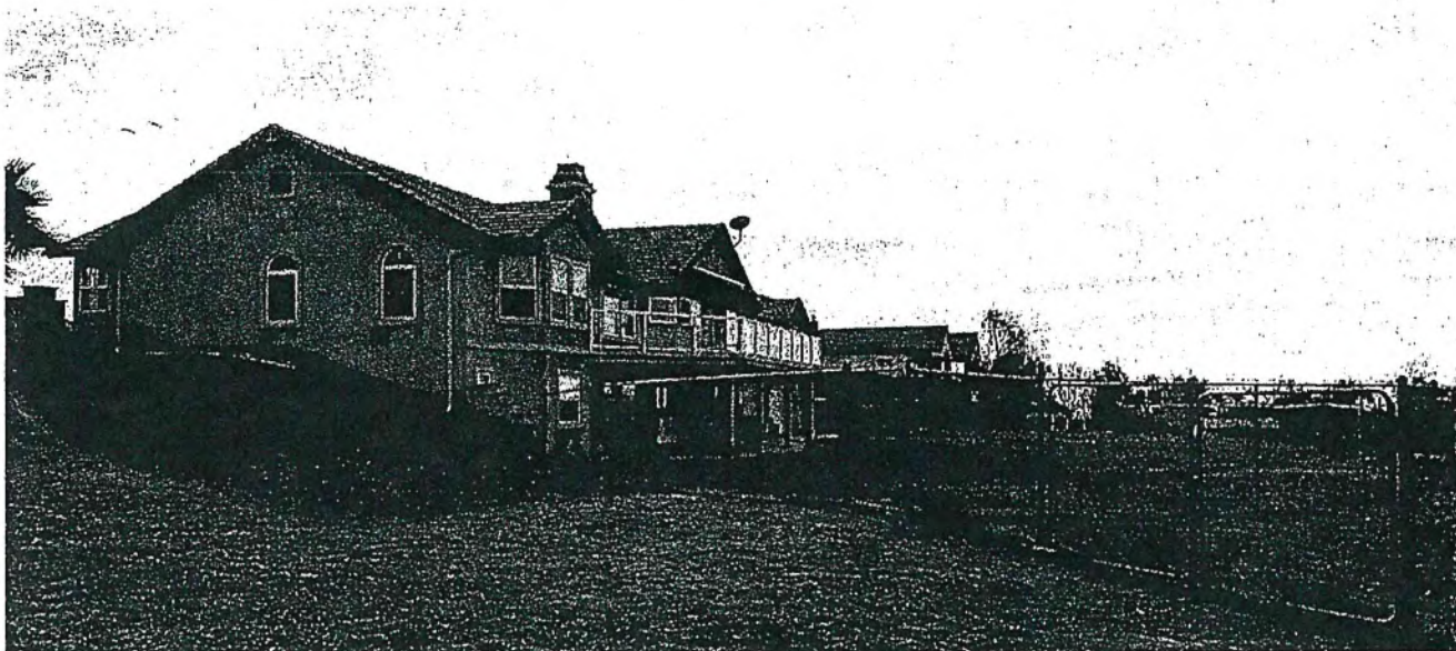
Yucaipa Ridge Road—use of slopes in development, single story front, two story back
