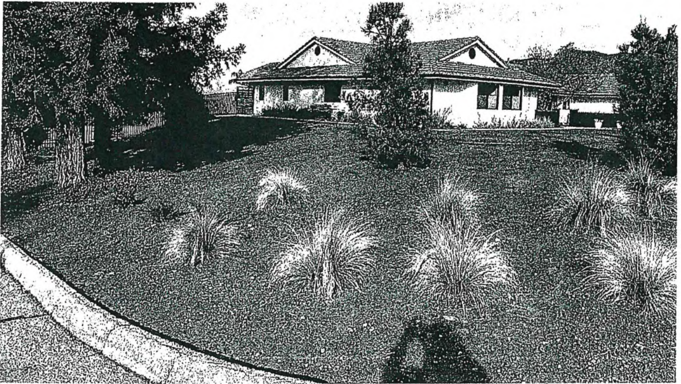
Yucaipa Ridge Road: Properties use slopes to advantage with flat slopes not exceeding 3:1 and generally much flatter
